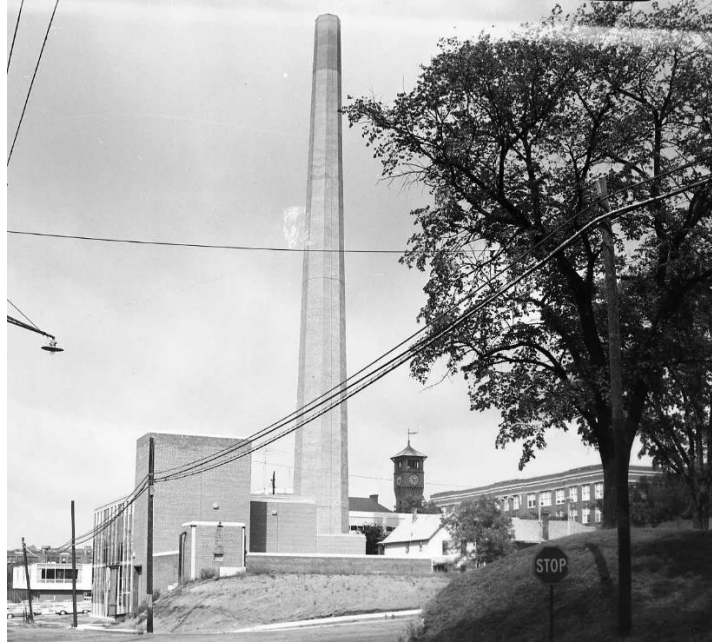
Figure 6. Photograph of heating plant. 1965. UW-Stout Archival Negative. 1965_244_002. University Archives, University of Wisconsin-Stout, Menomonie, WI.
