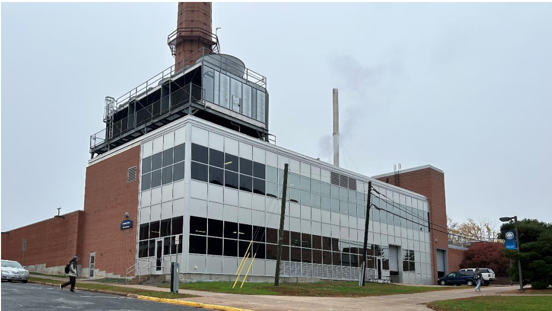
Fig 3. UW Stout Heating Plant in daytime. Photo by Author on 29 November 2023.
