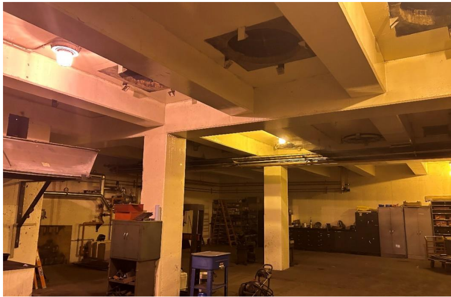
Fig 7. UW Stout Heating Plant old coal deposit room. Photo by Author on 29 November 2023.
