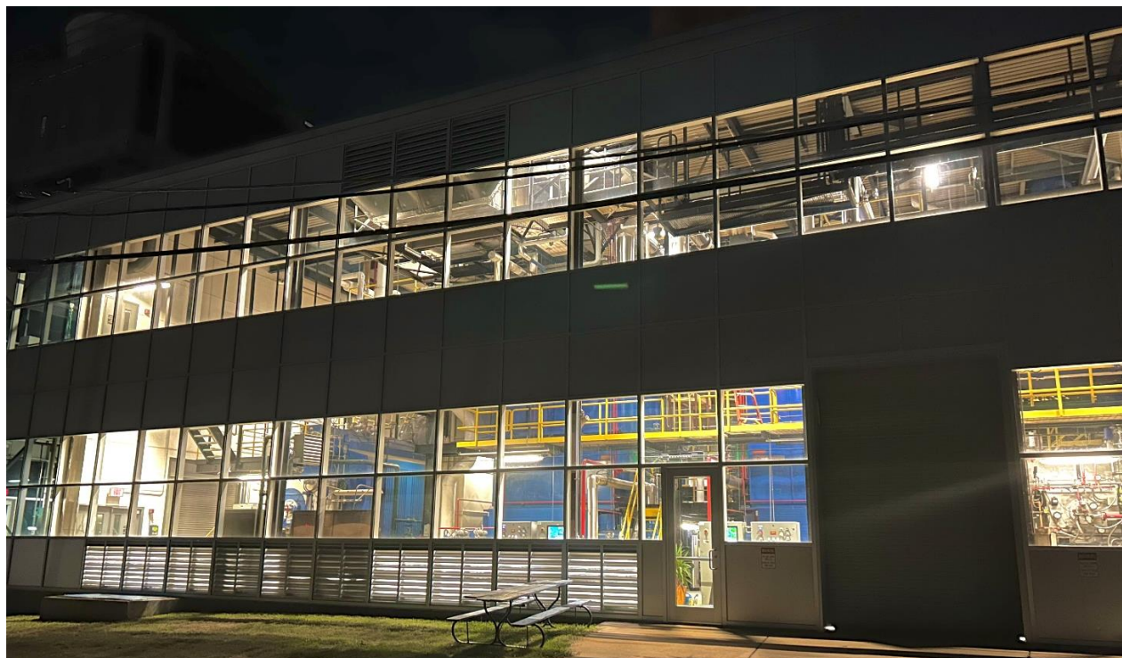
Fig 2. UW Stout Heating Plant at nighttime. Photo by Author on 2 September 2023.
