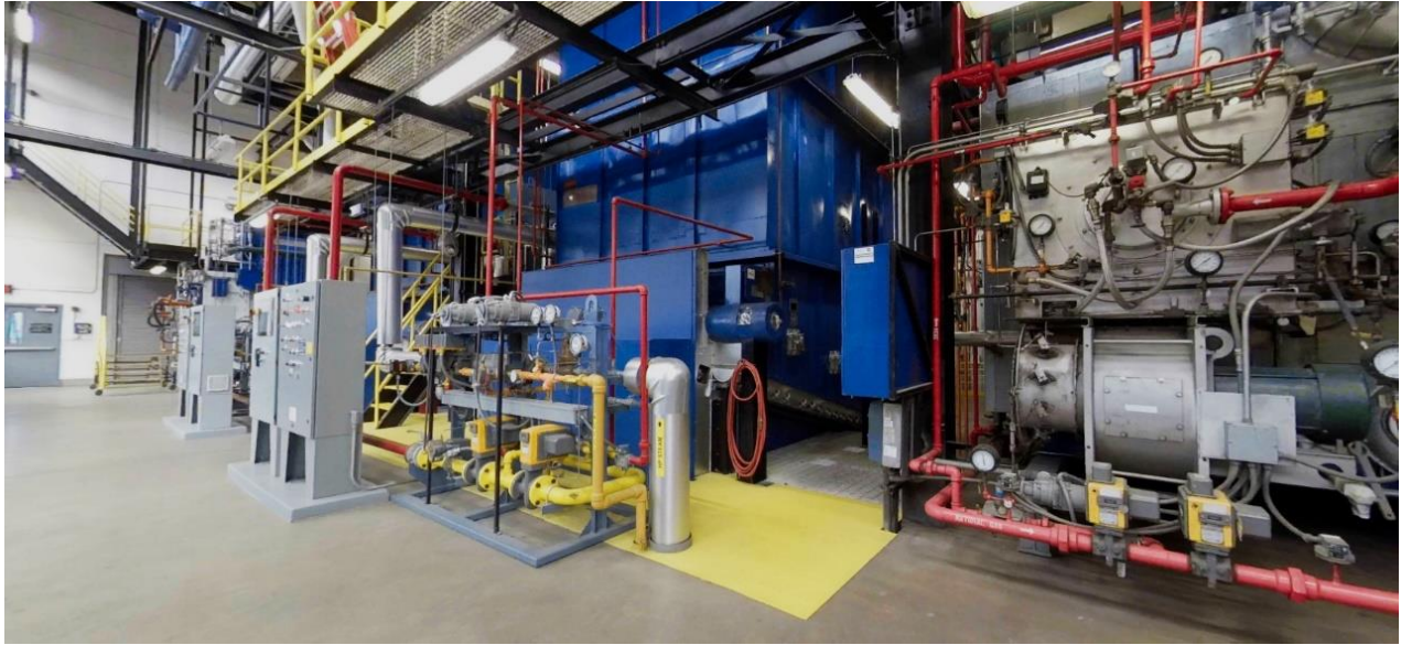
Fig 4. UW Stout Heating Plant boiler system. “Learning Opportunities.” Learning Opportunities | Thermodynamics Virtual Field Trip, uwstout.github.io/VirtualFieldTripStudy/infoPages/02-LearningMaps.html . Accessed 11 Dec. 2023.
