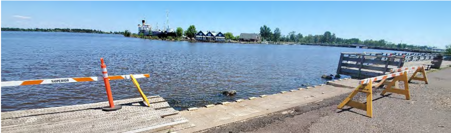
Image: Barricades indicate hazards after storm damage.
