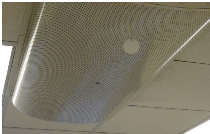
Figure 1: A glass fiber filter hanging from the air exchange in the chemistry lab.
