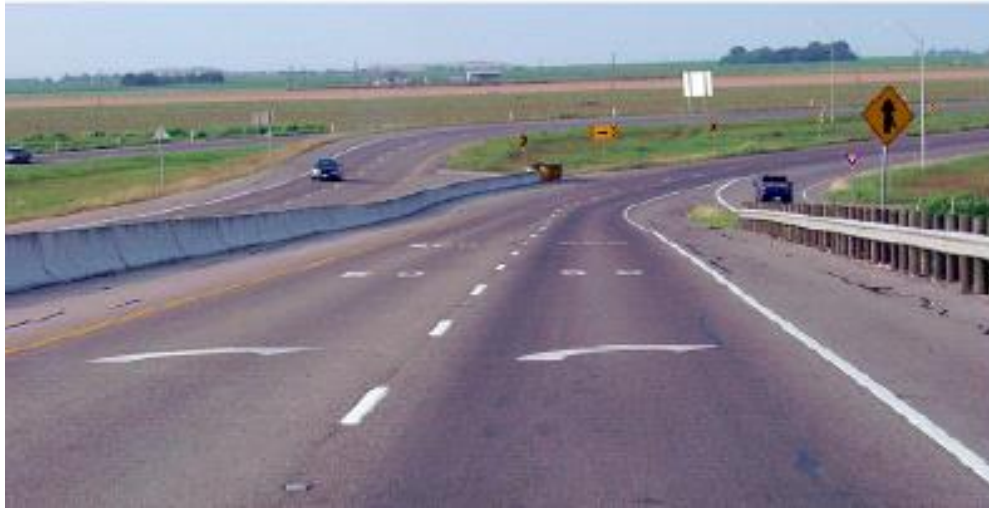
Figure 9. Curve Arrow and Advisory Speed Treatment on Urban Road (Chrysler and Schrock, 2005)
