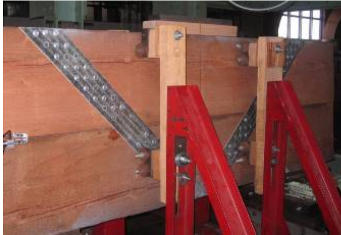
Figure 49: Two members from the depth series stacked and fastened in a V formation with FRP strips and screws. Each beam was 14" deep and the entire system was 28" deep. The FRP strips were 4" wide.
