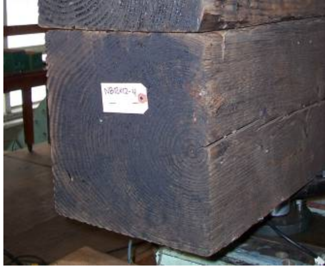
Figure 23: Full sized 12" x 12" creosote treated specimen.
