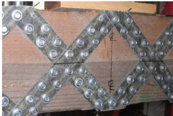
Figure 27: Two members from the width series stacked and fastened with FRP strips and screws.
