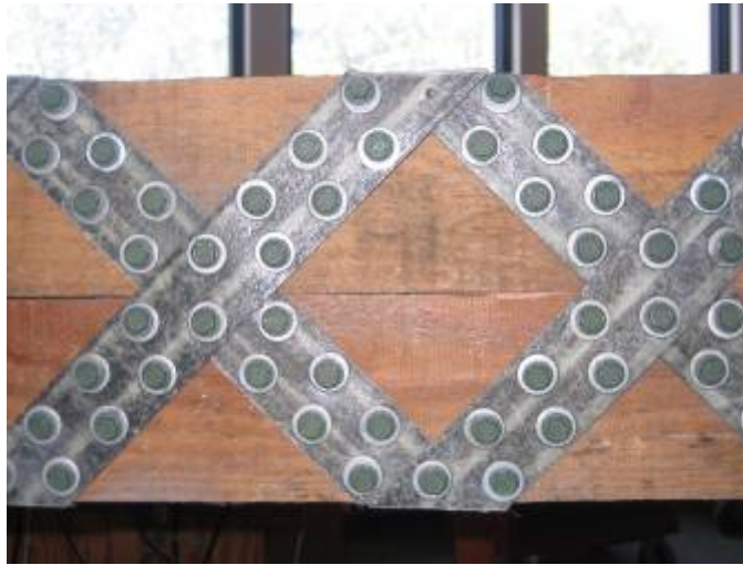
Figure 38: FRP X-braced specimen finished product. Each beam was 4” deep and the system was a total of 8” deep. Note a missing screw at the top where strips overlapped; in some cases the hole was too close to the edge of the beam and would cause splintering if drilled, or a knot in the wood prevented a screw from being placed.
