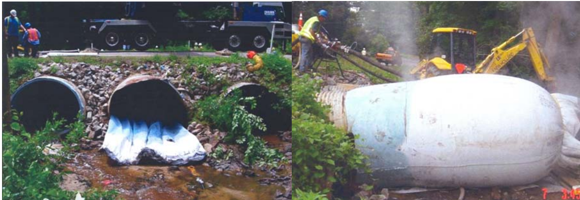
Figure 3-3 Pull and Inflate process (NASSCO, 2007).
