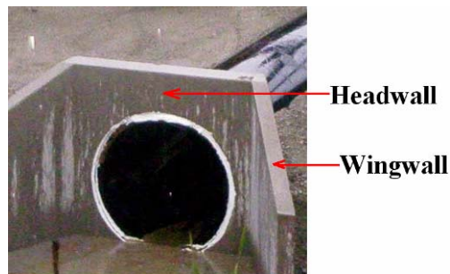
Figure 1-10 Culvert Showing Headwall and Wingwall
