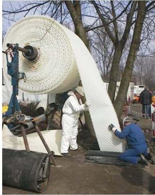
Figure 3-21 Insertion of the anchored liner (ASCE, 2008).
