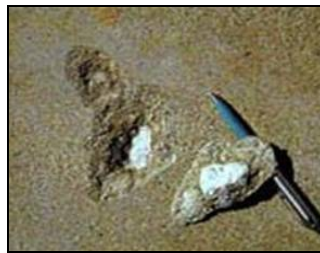
Figure 2-11 Pop-outs in a Concrete Structure. (Source: Concrete Sealers, Specialty Coatings and Consulting, 2006)
