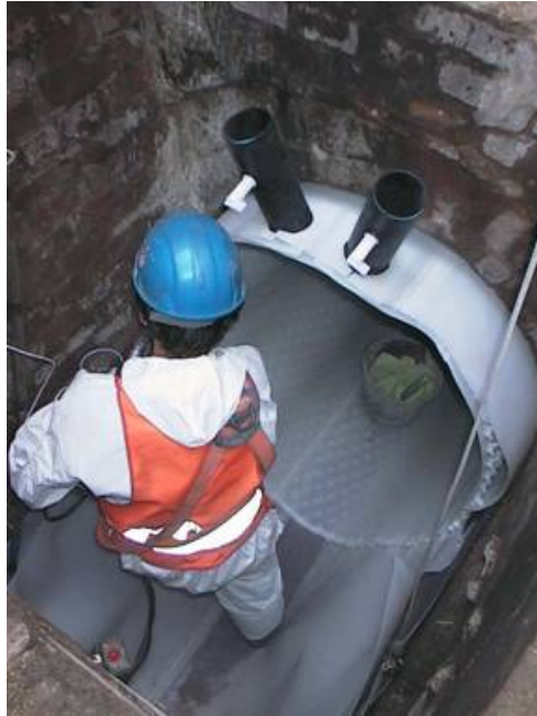
Figure 3-23 Attachment of grouting ports (ASCE, 2008).
