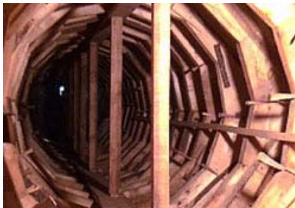
Figure 3-25 Installation of form works in preparation for grouting (ASCE, 2008).
