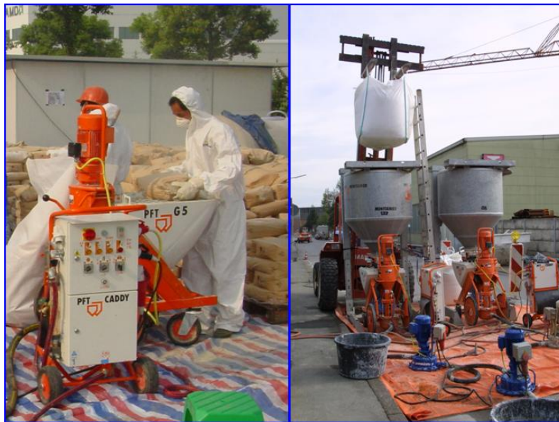
Figure 3-26 Small scale and large scale grout mixing set-ups (ASCE, 2008).
