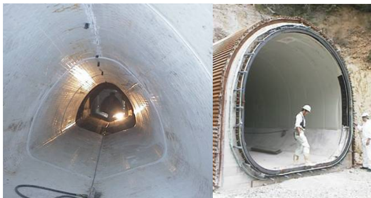
Figure 3-20 Using of FIPP in different culvert shapes (ASCE, 2008)
