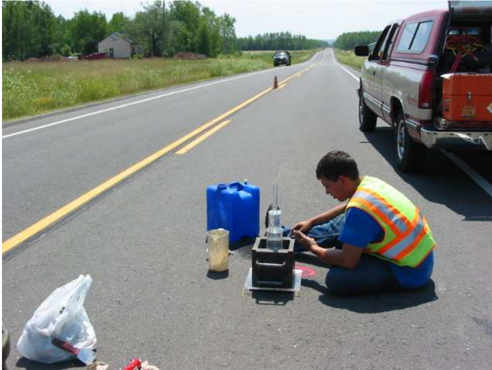
Figure 4.3 Measuring Falling Head in NCAT Water Permeameter
