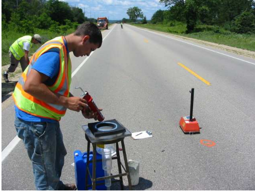
Figure 4.1 Applying Sealant to Rubber Gasket for Water Permeability Test
