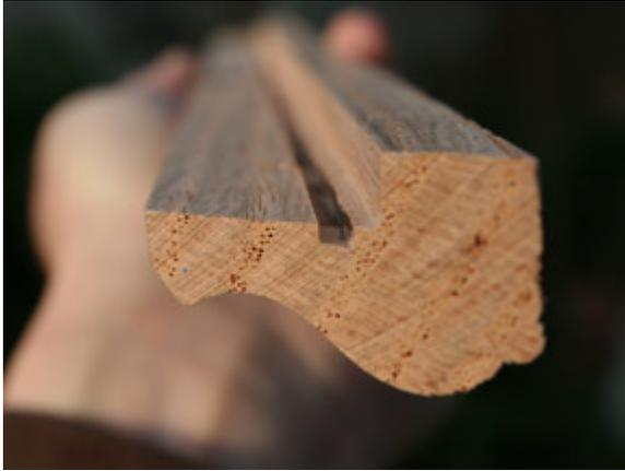
Figure 4.2: Channels added for running wires
