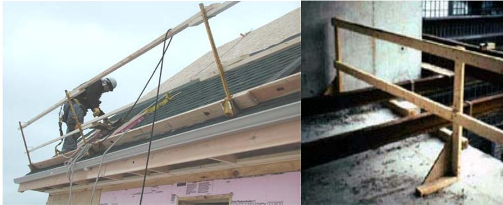
Figure 1.4: Guardrail (Acro Building Systems and OSHA)
