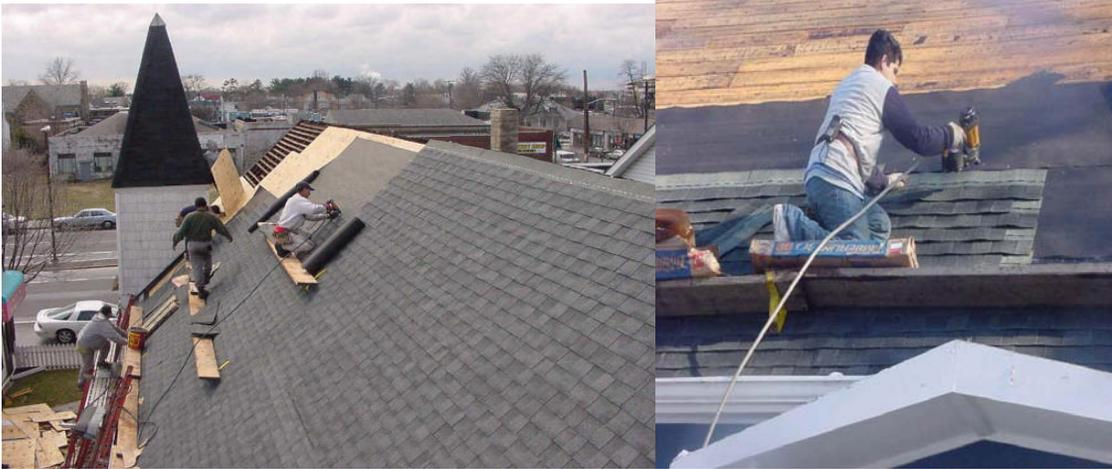
Figure 2.1: Slide guard (Roofer 911).
