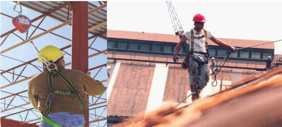
Figure 1.3: Personal Fall Arrest System (Acro Building Systems)
