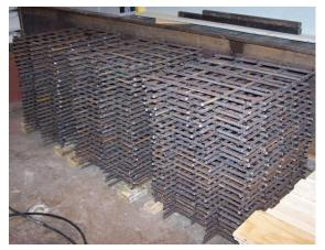
Figure 43: Layers of prepared reinforcement
