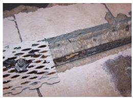
**Figure 134:** Close-up of TSZ w/EP-C(2) exposed rebar
