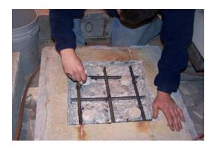
**Figure 67:** Application of anti-corrosion coating to reinforcing steel
