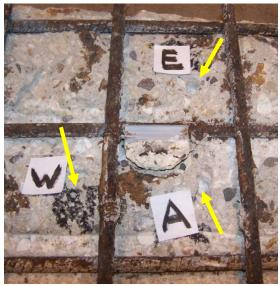
**Figure 88:** Location of "near anode" chloride tests for EA-B
