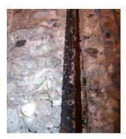
Figure 118: Close-up of TSZ(2) exposed rebar
