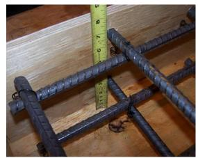
Figure 44: Clear cover to reinforcement
