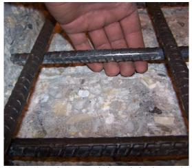
**Figure 60:** "Finger-gap" below reinforcing steel
