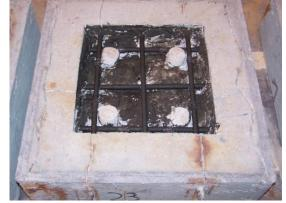
**Figure 68:** Application of bonding agent to substrate (not applied on or directly below anodes)
