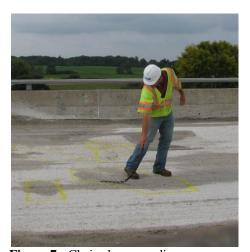
Figure 7: Chain-drag sounding
