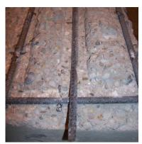
**Figure 198:** Close-up of T-SS(2) exposed rebar
