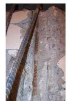
Figure 214: Close-up of EP-C exposed rebar
