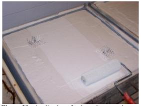
**Figure 38:** Application of polyurethane coating to epoxy coating
