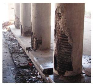
Figure 5: Spalling of concrete
