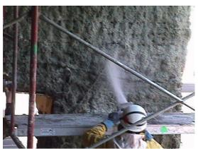
Figure 23: Application of cellulose fibers (91)
