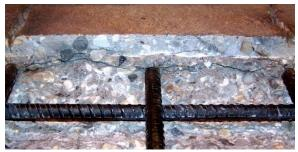
Figure 4: Delamination of concrete
