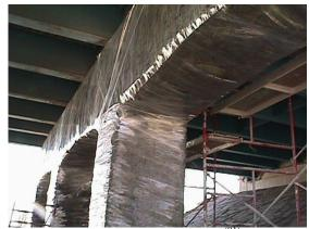
Figure 24: Operational ECE system <sup>(9)</sup>
