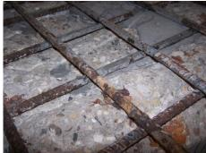
**Figure 242:** Close-up of Control(1) exposed rebar after 6-months
