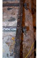
**Figure 230:** Close-up of Control(2) exposed rebar
