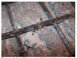
**Figure 166:** Close-up of EA-A(2) exposed rebar
