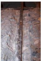
Figure 206: Close-up of A-C exposed rebar
