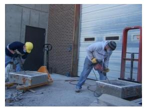
Figure 57: Concrete removal
