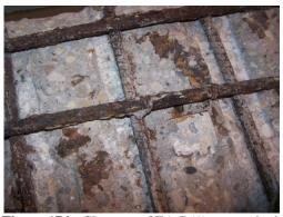
**Figure 174:** Close-up of EA-B(1) exposed rebar
