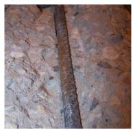
**Figure 190:** Close-up of T-SS(1) exposed rebar
