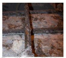
**Figure 182:** Close-up of EA-B(2) exposed rebar
