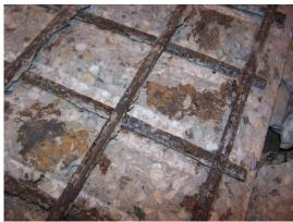
Figure 222: Close-up of Control(1) exposed rebar
