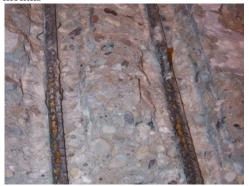
**Figure 110:** Close-up of TSZ(1) exposed rebar
