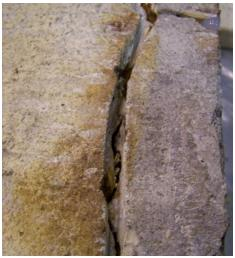
**Figure 63:** Presence of cracking exposed through routing
